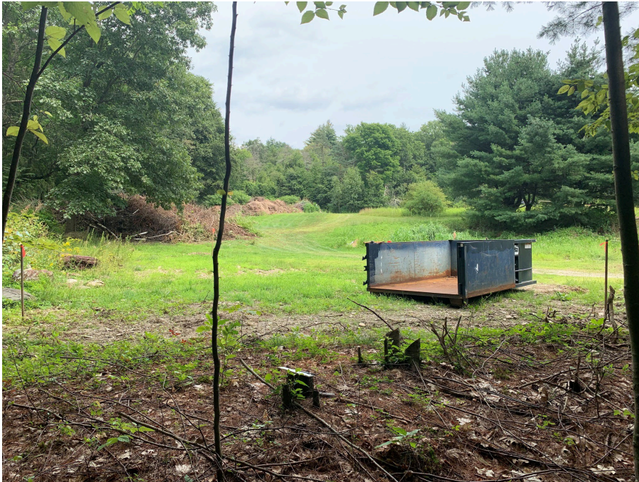
View of the staked 33' x 40' proposed maintenance building footprint, looking due east.
