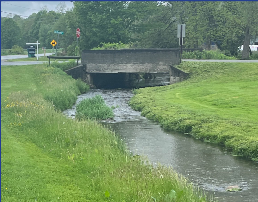
Downstream Bridge Fascia (Looking Upstream)
