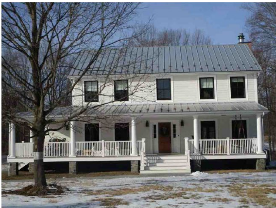
Home has new windows, Hardie board siding, a metal roof with decorative snow guards
