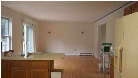
Family Room before renovation
