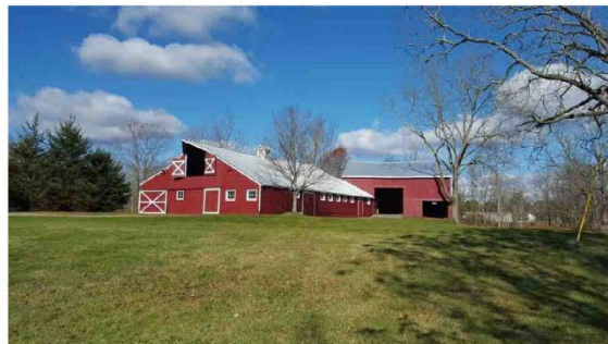
Barn after renovations. Aside from interior improvements, a new metal roof was installed on the barn
