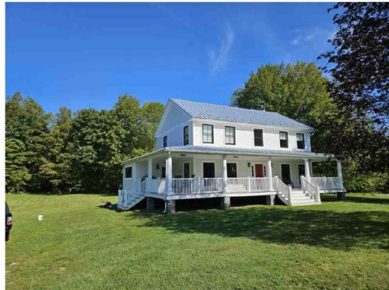
After renovations with new wraparound porch, Hardie board siding and metal roof with decorative snow guards
