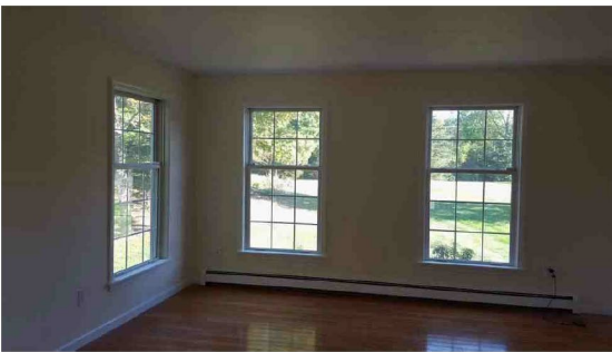
Living room before renovation
