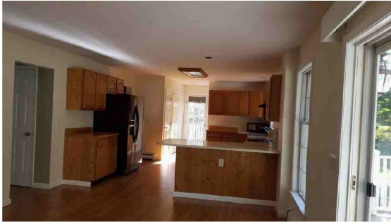
Kitchen before renovation
