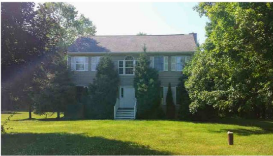
Before renovations with stock windows and asphalt roof
