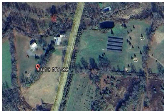
After solar panels
