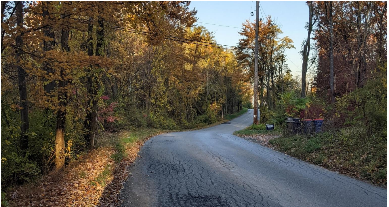
Figure 6: Stanford Rd. view north/ northeast of Clear property - Barto property driveway
