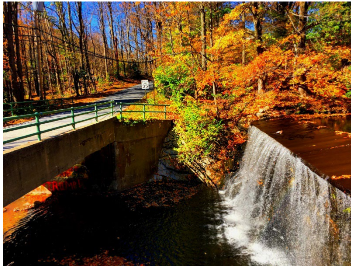
Photo 11. Culvert on Stanford Road, Washington (Beatrice Moritz)
