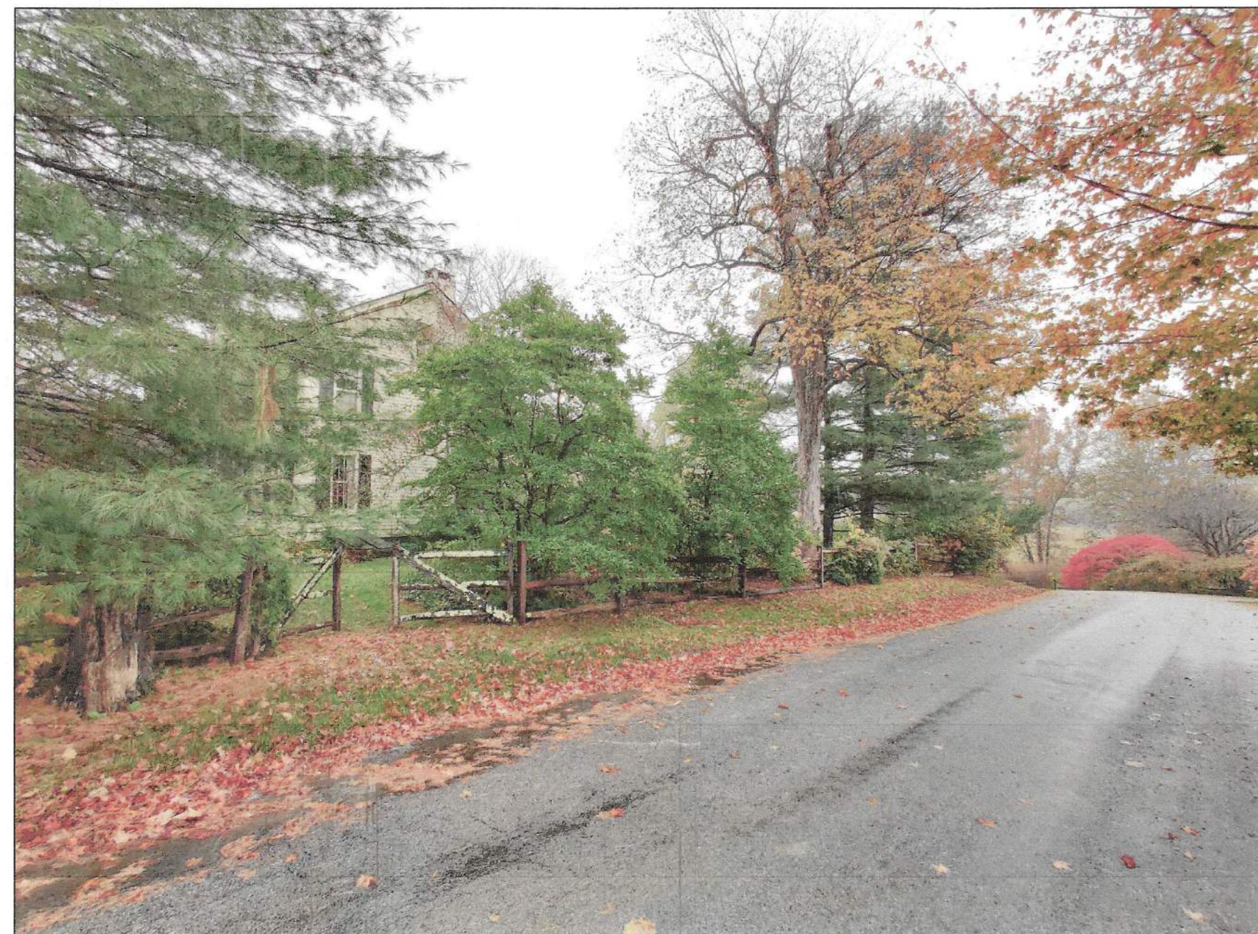
LOOKING SOUTH AT SIDE OF HOUSE FROM FOWLER ROAD
