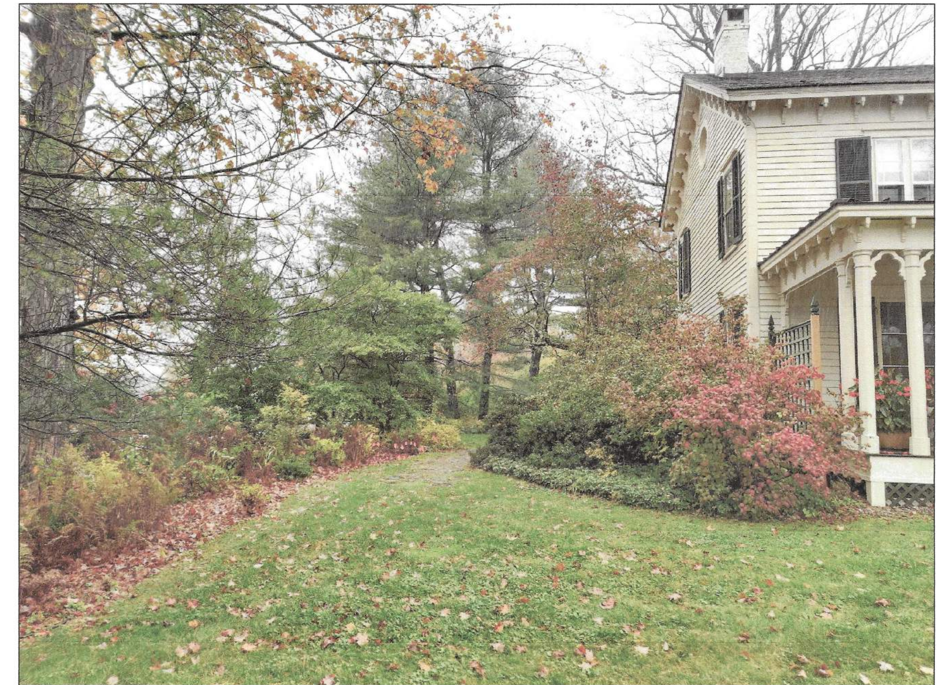
LOOKING NORTH FROM REAR OF HOUSE
