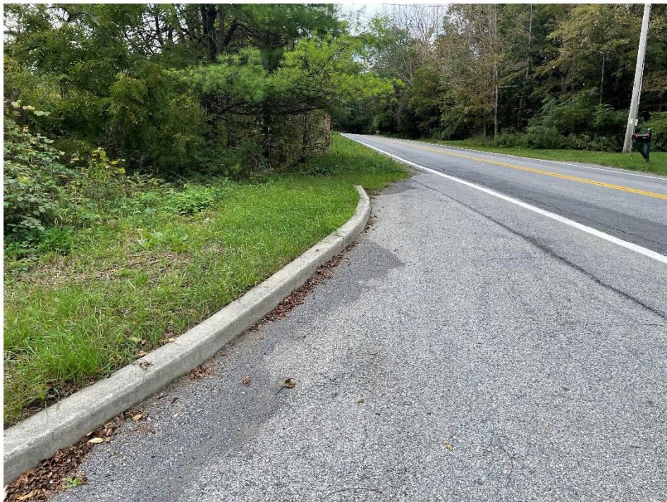
South curb cut brush/tree growth removed. Full view of traffic to south before intersection.
