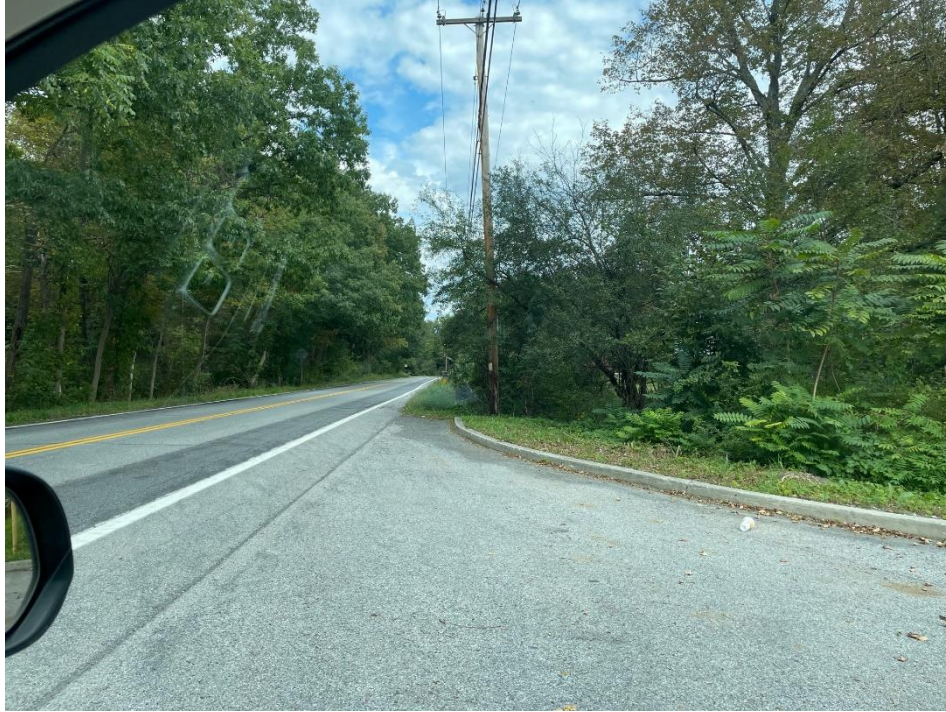
Unimpeded view to north approaching intersection.
