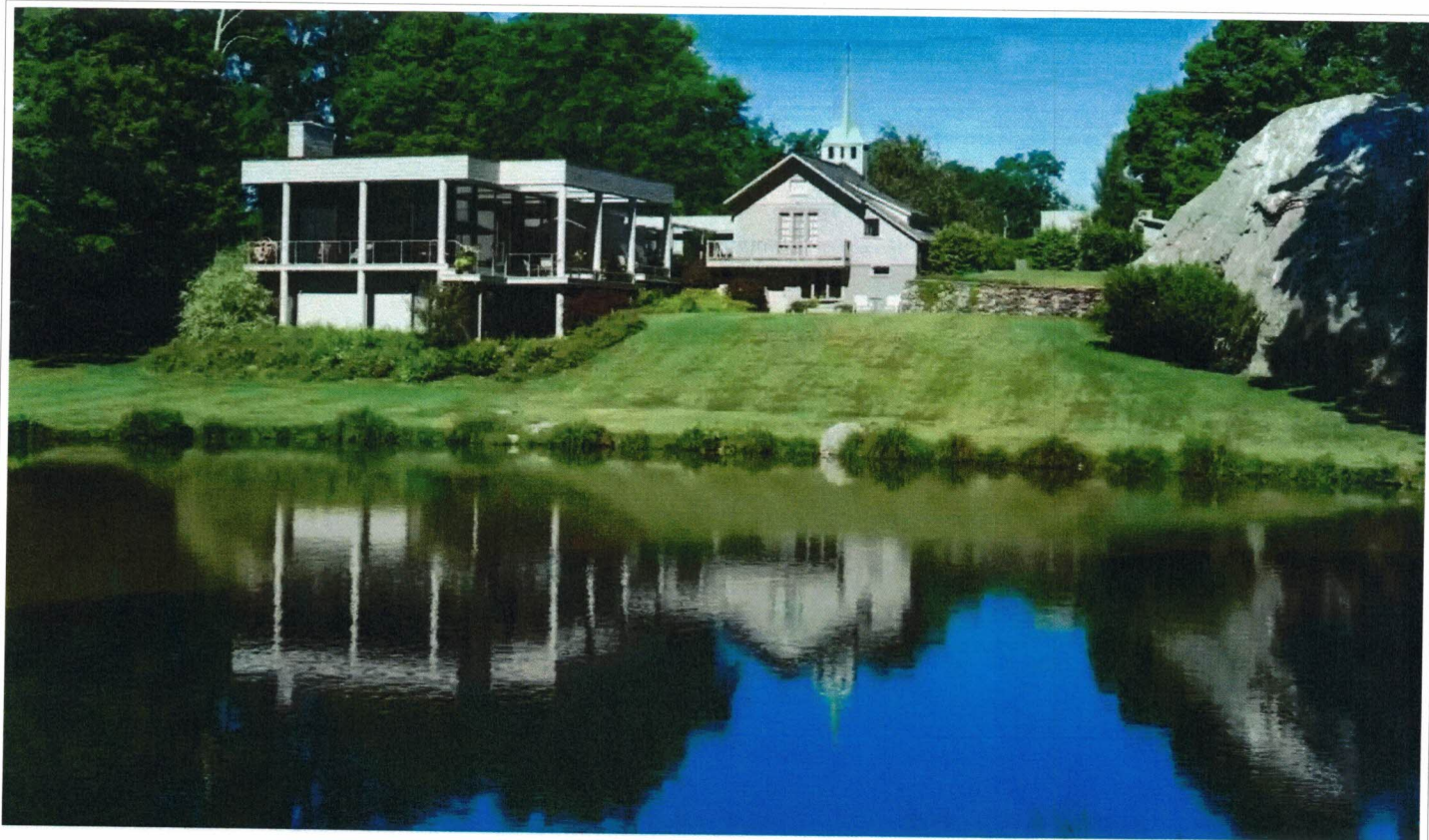
Area 1: Existing - shown almost all the present building to be within the 100-foot buffer
